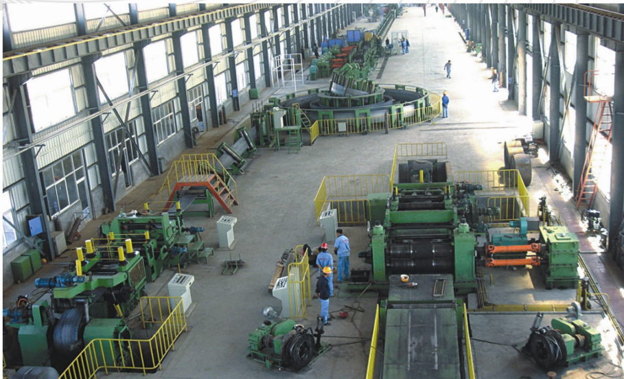
大直径高频焊管生产线全景 (large diameter high frequency welded pipe line)
